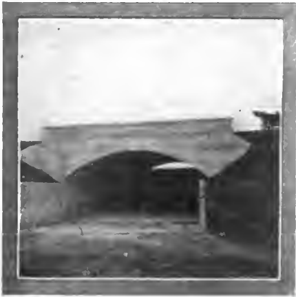
Side view of one of the arches over a "fill"
